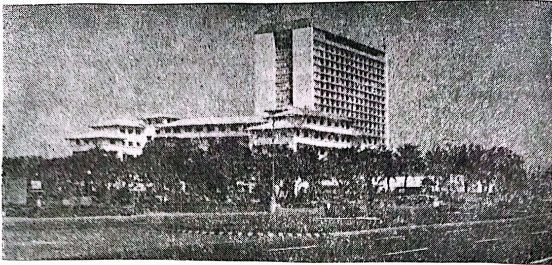
FIG. 6. THE MANILA HOTEL IS LOCATED ADJACENT TO THE PORT DISTRICT, AND DATES FROM THE ERA WHEN TOURISTS ARRIVED BY SHIP.
